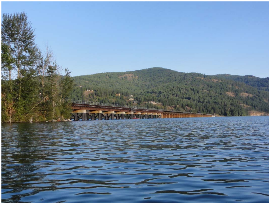
Key View 4a: Existing Bridge 3.9 from the north shoreline of Pend Oreille River.
